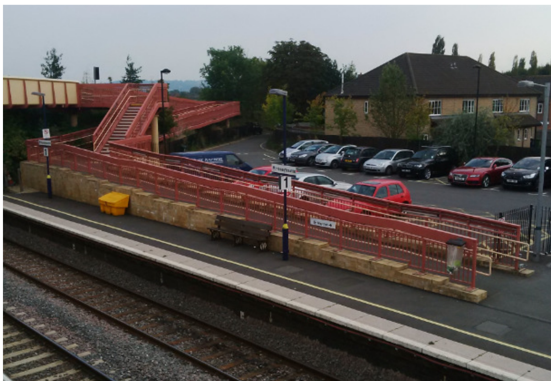
Figure 15: Honeybourne (Category B) – does not meet new-build standards, but the station is considered usable by many people who need step-free access
