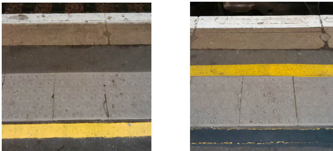
Figure 23: At West Croydon Network Rail has specified Platform 1 (left) but TfL has specified Platform 3 (right). The two platforms are adjacent sides of the same island, with the obvious potential for confusion
