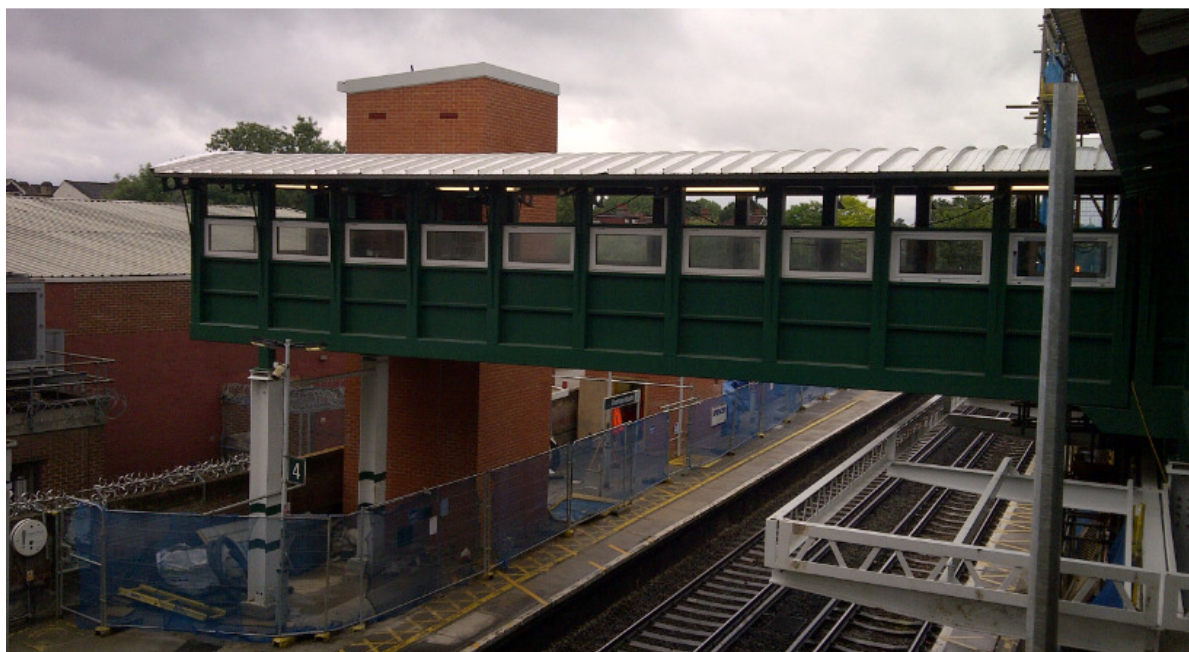
Figure 12: Access for All lift scheme under construction at Thornton Heath
