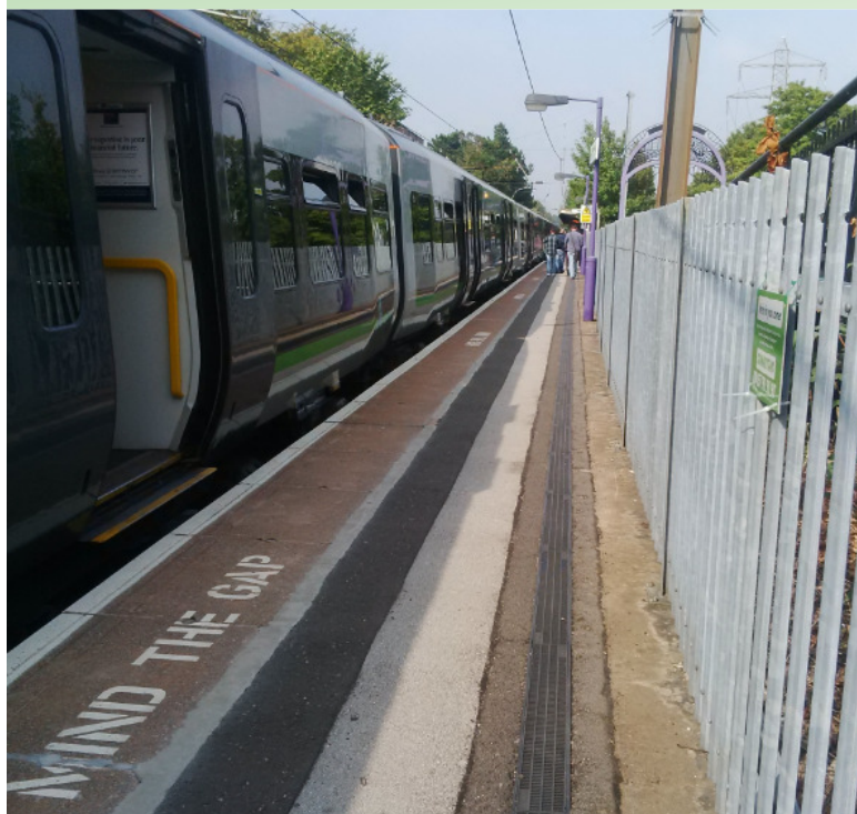
Figure 20: Narrow section of platform at Bournville
