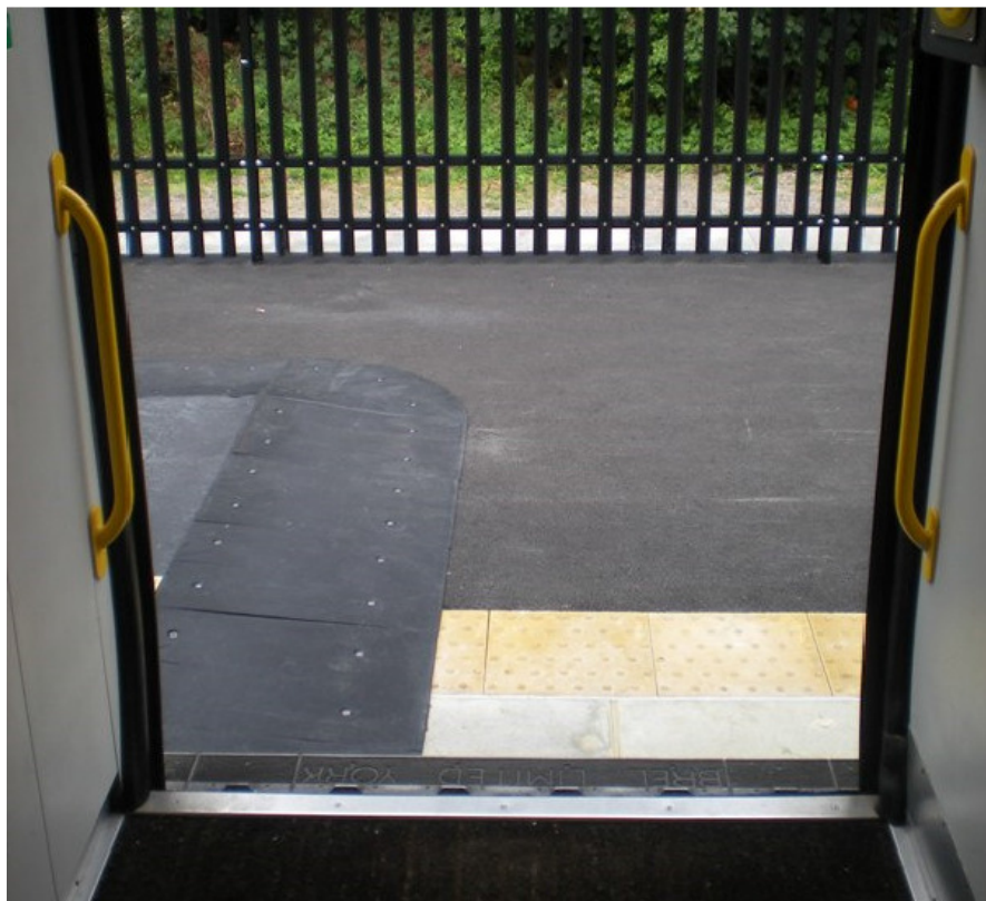
Figure 21: At St Albans Abbey the Hump does not line up with the wheelchair-accessible doorway – passengers may step down onto a sharply-sloped area
